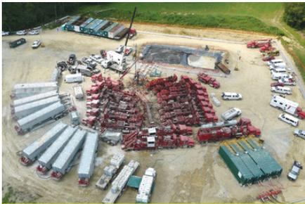
Hydraulic fracturing has been used to produce oil and natural gas since 1949. The process involves pumping a mixture made up of 99.5% water and sand, and a minimal amount of additives, into the ground under high pressure. The solution opens tiny fractures in the rock to allow a pathway for the oil and gas to enter the wellbore. It typically takes about a week to complete a hydraulic fracturing operation.
